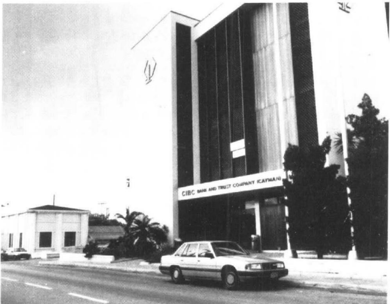
Two of the numerous banks located in the Cayman Islands Courtesy Warren Yeager
